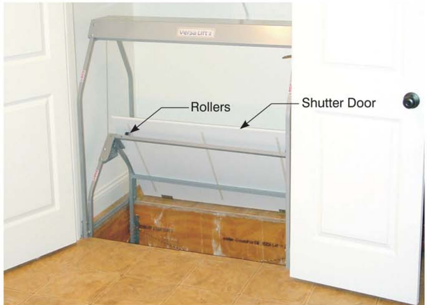
Fig. 2: As the lifting platform descends, rollers lower the shutter door.
